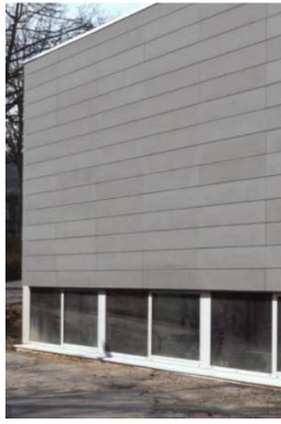
Fig. 4 - TRC applications - façade RWTH Aachen University (Germany). Source: [1].
