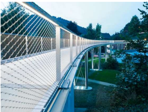
Fig. 6 - TRC applications - bridge in Albstadt-Lautlingen (Germany). Source: Innovation in Textiles by Groz-Beckert KG.
