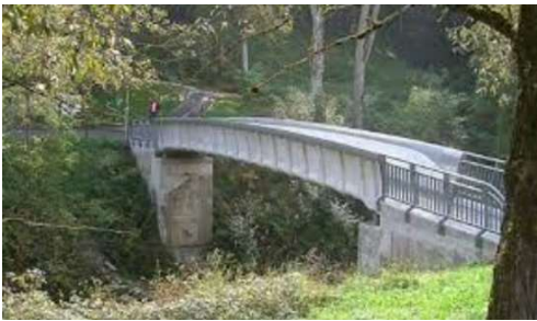
Fig. 5 - TRC applications - bridge in Kempten (Germany). Source: [7].
