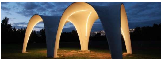
Fig. 7 - TRC applications - pavilion at TU Chemnitz (Germany). Source: [8].
